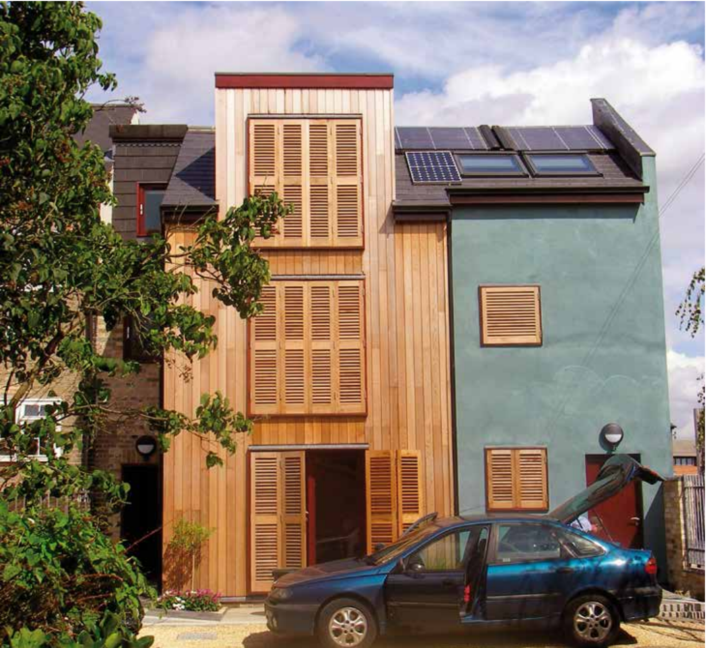
Figure 6 External shutters may become a necessary addition in the UK. Image courtesy of AC Architects.
